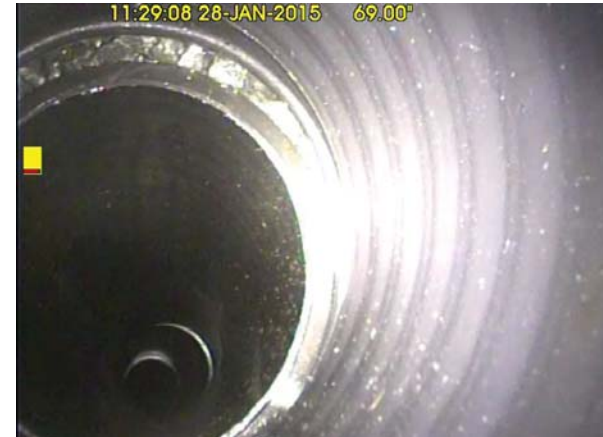
Figure 3-18. Offset Joint, a Defective Displacement of at Least One Pipe Thickness at a Joint.
