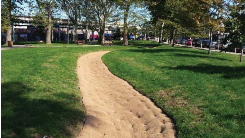
Figure 2-3. Example of Erosion Control
