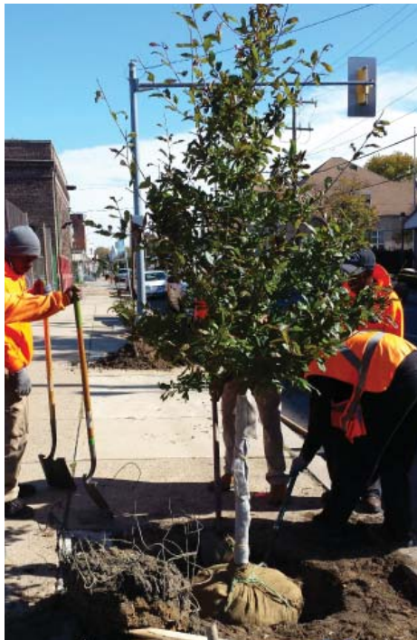
Figure 2-11. A Tree Being Planted
