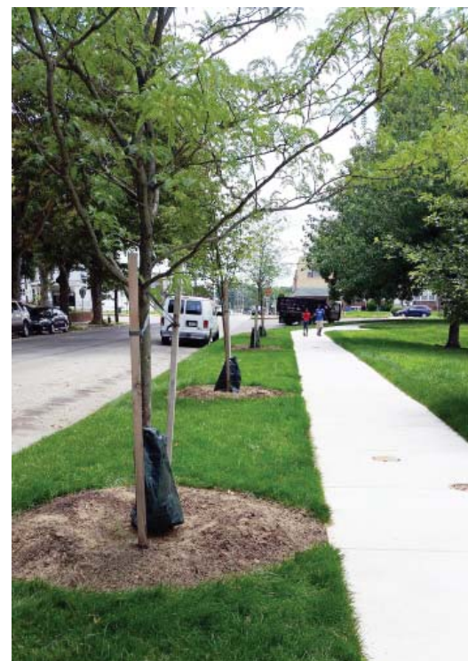
Figure 2-12 Gator bags installed on trees
