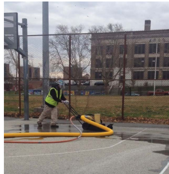
Figure 4-2. Pressure Washer with Vacuum Attachment
